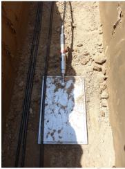
Figure 5. Installation of earth stress sensor [8].
